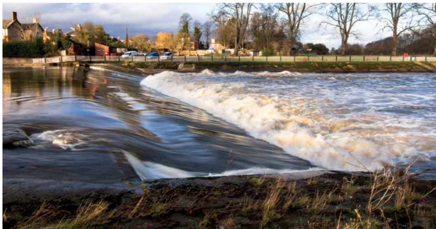
Even in high low conditions the smooth water above the weir can appear relatively benign. However the boil line and recirculation can clearly be seen on this weir on the River Severn, UK.
